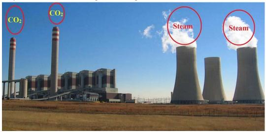
This picture shows so called greenhouse gas emissions of CO<sub>2</sub> and water vapour from a U.S. coal fired power plant.
