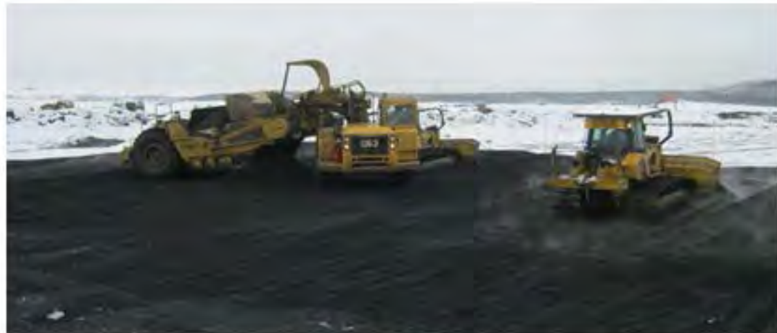
Photo of a CAT 631E dumping and spreading coke at the edge of a pond road
