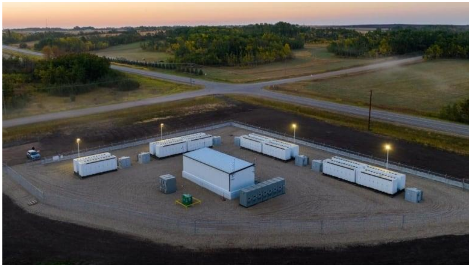
Enfinite's eReserve3 facility, in the Hamlet of Clairmont in the County of Grande Prairie, is one of nine battery-storage facilities the company has connected to Alberta's electricity grid. Each facility has a 20 MW, 35MWh capacity. (Submitted by Enfinite)
